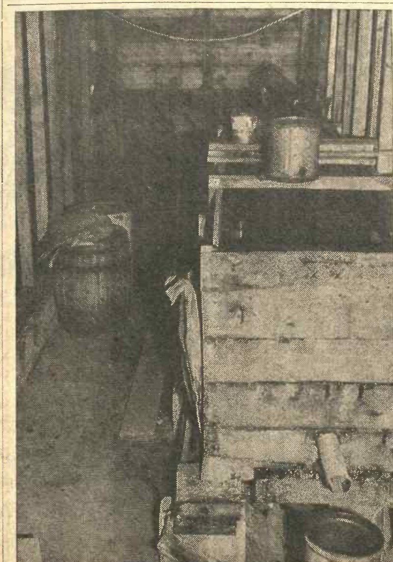
CONDENSER & SPOUT —In this aisle is shown the condensers. The one in the foreground was approximately 5 ft. wide by 4 ft. high by 24 ft. long. It was filled with water in which the worm was submerged, connected to the spout in front. Whiskey, as it came from the still, poured into a five gallon paint can.
